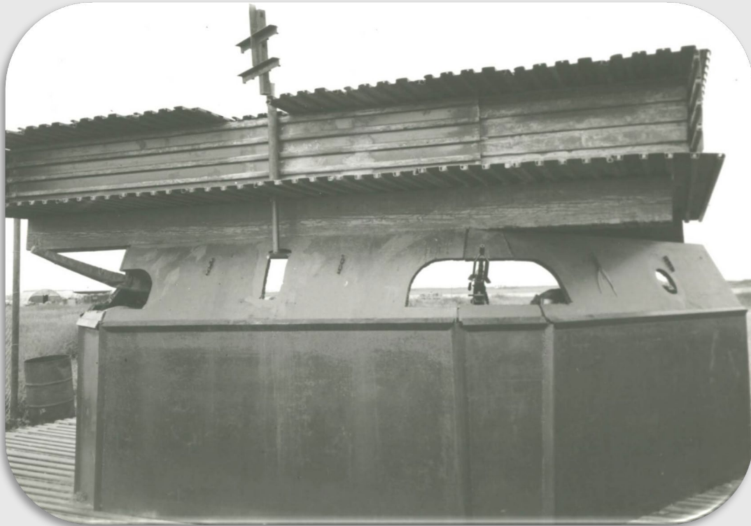
Bunker at Tan Son Nhut, ca. 1960s (USAF Photo)
